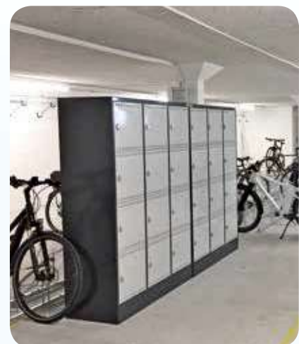
E-compartment cabinet as e-bike charging station
